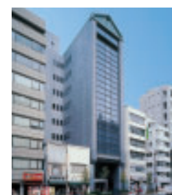
KODONMACHI SHIN-NIHONBASHI BUILDING
