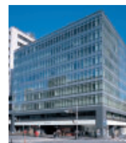
SANNO GRAND BUILDING
