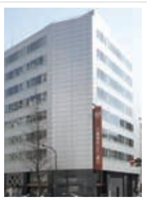
A-40 虎ノ門東洋ビル Toranomon Toyo Building
