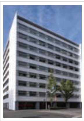
A-53 KDX博多南ビル KDX Hakata-Minami Building
