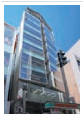
A-45 KDX六本木228ビル KDX Roppongi 228 Building
