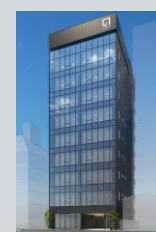
S-GATE FIT 八丁堀
