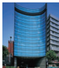
I-33 IKEBUKURO YS BUILDING 池袋YSビル
