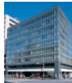
SANNO GRAND BUILDING
