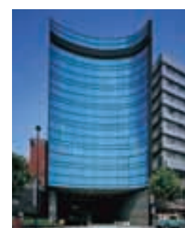
I-23 IKEBUKURO YS BUILDING 池袋YSビル
