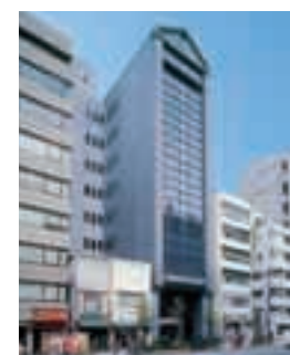
KODENMACHO SHIN-NIHONBASHI BUILDING
