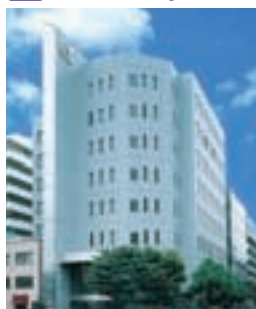
Of -06 NV富岡ビル NV Tomioka Building
