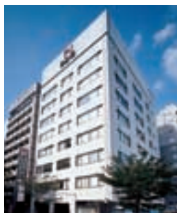
Of -10 日総第15ビル Nisso Dai 15 Building
