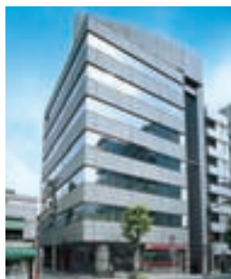
Of -12 八丁堀SFビル Hatchobori SF Building
