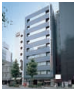
Of -14 KCAビル KCA Building
