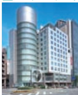
Of-03 三宮三和東洋ビル Sannomiya Sanwa Toyo Building
