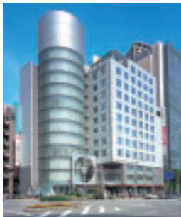
Of-19 三宮三和東洋ビル Sannomiya Sanwa Toyo Building
