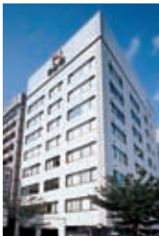
Of -10 日総第15ビル Nisso Dai 15 Building
