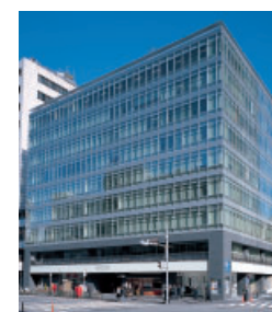
SANNO GRAND BUILDING
