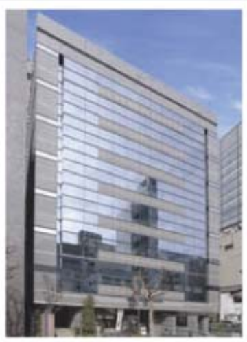
A-15 KDX浜町ビル KDX Hamacho Building
